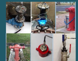
Typical sensing installation alternatives on existing hydrants, pipe taps or air valves
